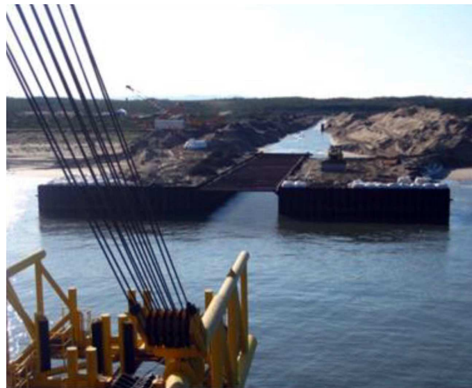
Fig. 10.2-4 Cofferdam for pulling of pipeline on shore at the Kirinskoye field, Sakhalin Island
