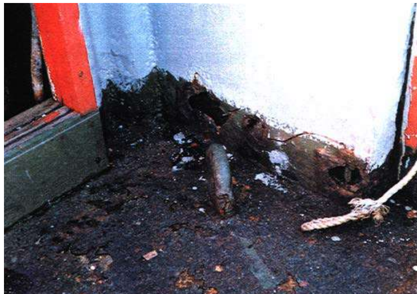
Photograph 1 Corroded accommodation house structure
